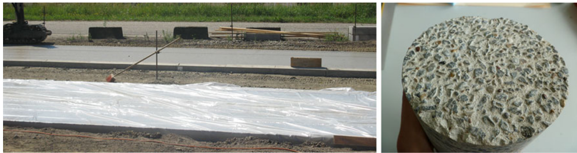
Fig. 11 Trial section of double layered concrete with \text{TiO}_2 in the top layer on industrial zone “Den Hoek 3” in Wijnegem
