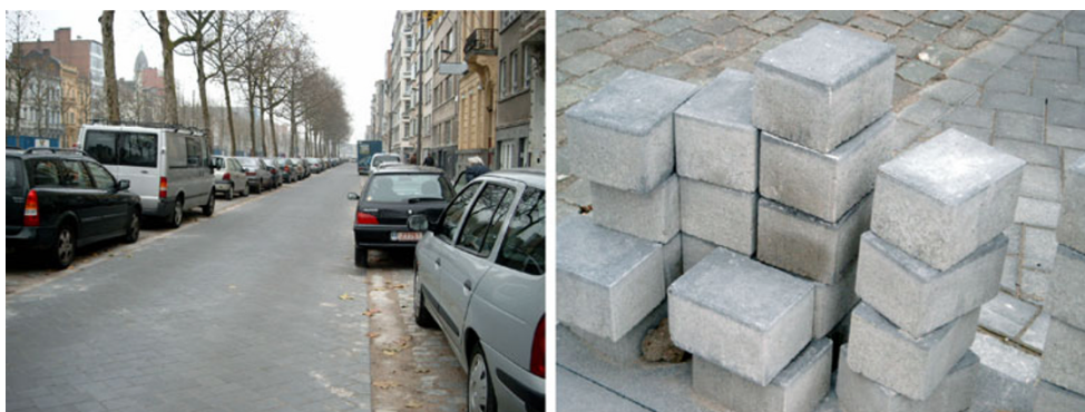
Fig. 5 Separate parking lanes at the Leien of Antwerp with photocatalytic pavement blocks
